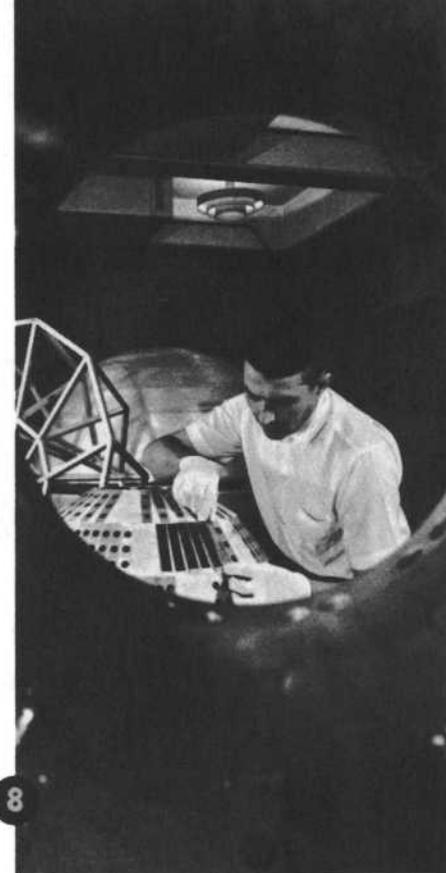
8 Finally, the cells are attached to the satellite. Internal conductors carry current to storage batteries, which in turn power the satellite's radio receiver and transmitter.
