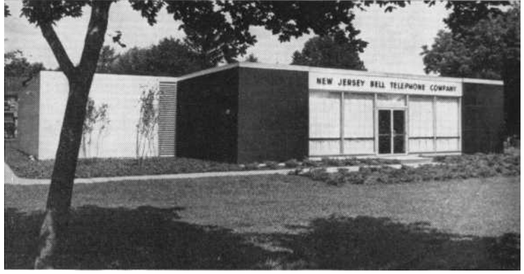
The Bell System's first commercial electronic central office is housed in this building at Succasunna. It began serving 4300 New Jersey Bell Telephone Co. customers on Sunday, May 30, 1965.
