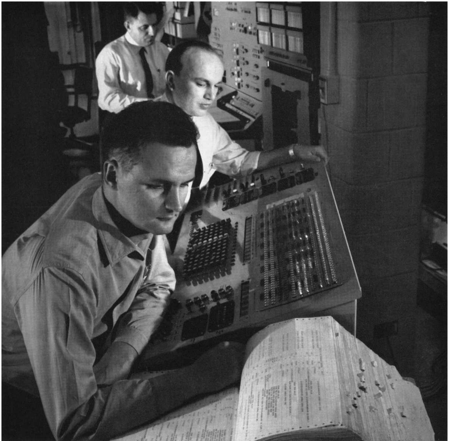
H. C. Przybysz, R. K. Voss, and T. E. Jackson (front to back) use the Central Control Manual Tester to test the No. 1 ESS installed for the C. & P. Telephone Co. at Chase, Maryland. The large book in the foreground contains program listings which are used to interpret the displays on the Tester lamp panels.
