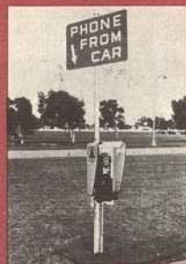
Walk-up and Drive-up Public Telephones provide service along highways, in parks, shopping centers.
