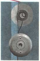
Cover plate for concealed wiring installed when home is built.
